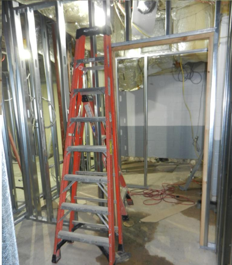
The floor has been filled with concrete and the wall studs are going up. Above is the Men's Room looking out toward the Auditorium. To the right is the front ADA Restroom looking back toward the second restroom in the former dish washing area..
