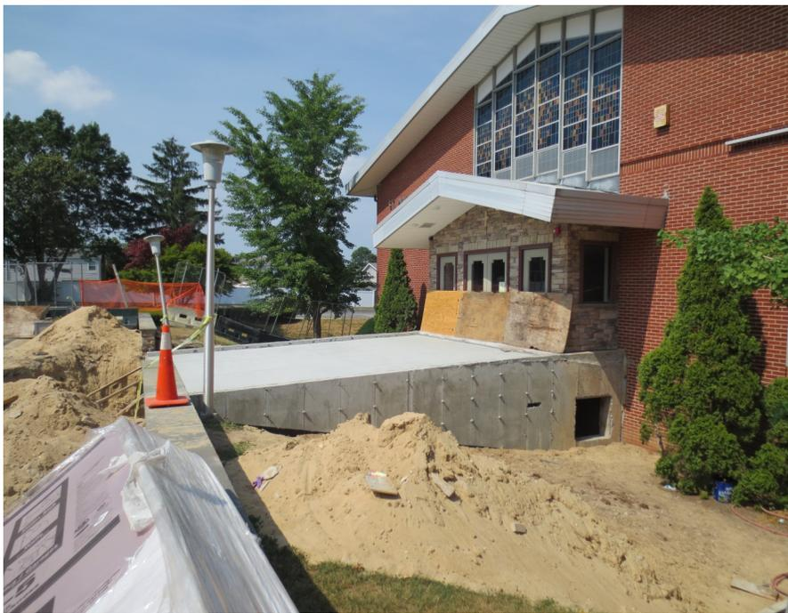
On Monday, the base concrete for the bridge deck was poured over the steel deck. The weather was perfect and there were no problems. As of today (Tuesday) we await the backfilling of the hole where the new sidewalk with wheelchair access will stand (lay?). Installation of the insulation and wirework for the for the ice melting system should be evident as you attend today.
